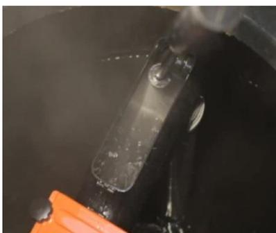
Alternatively, the filter strainer can be removed and cleaned manually. In doing so, it is important to clean the filter collection area with a high pressure cleaner or hose, to flush all dirt out through the emergency overflow before removing the strainer. In this way, the clean strainer can be re-installed without dirt and sludge fouling the lateral support guides to ensure a perfect re-insertion.
