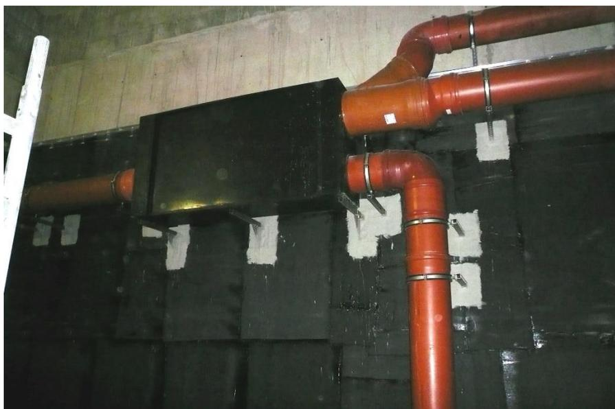
**DN300 Installation – Note approach piping not as recommended**
