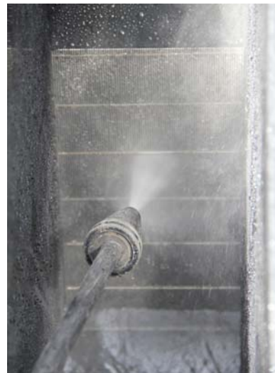
Fig. 16: Automatic cleaning with high pressure cleaner
